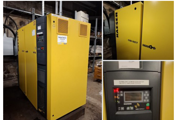
KAESER CSD 105 T SFC screw compressor, Erasteel Vikmanshyttan
