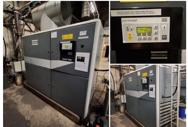
ATLAS COPCO GA50VSD screw compressor, Erasteel Vikmanshyttan
